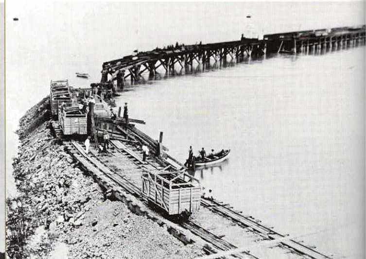
The Gulnare Jetty after damage caused by strong erratic tides and borers in 1893 (Tracey Collection, NT Library)
